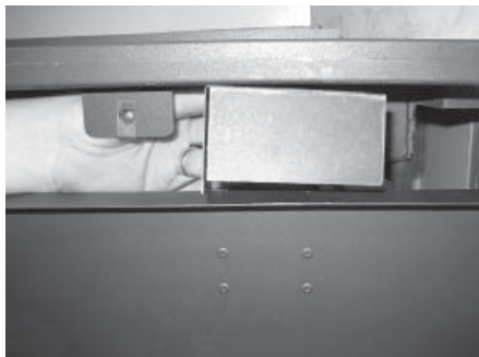
DC Spark Box Bracket Assembly partially removed.
