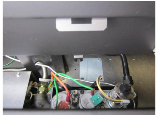
**NOTE:** Use pliers to adjust the air shutter (it will be hot). Typically, the air shutter is more closed (right) on NG, more open (left) on LP.
