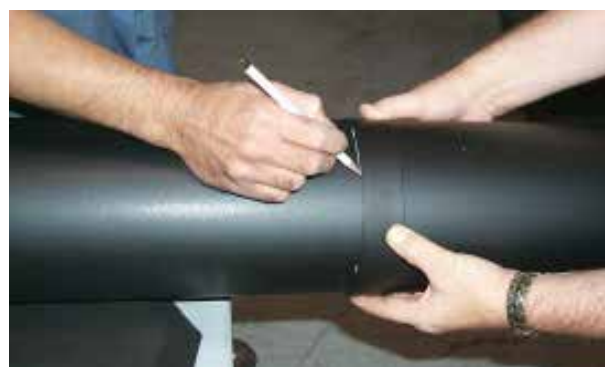
Use trim collar as a guide to 'connect the dots'.
