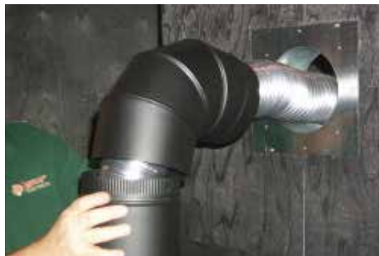
Slide 90° elbow over flex
