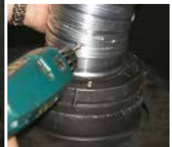
Fit flex over adaptor and secure with Mill-Pac and 3 screws.
