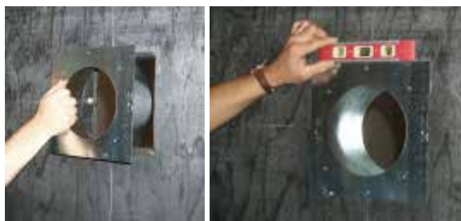
Wall Thimble - level & secure with 4 screws.
