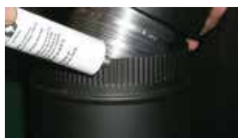
Secure 90° elbow to vertical pipe with Mill-pac and 3 screws.
