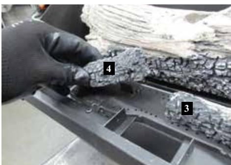
Log 4 rests against tab on burner
