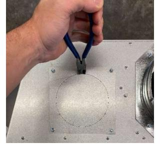
8 Grab on to the knockout with pliers and bend it back and forth until the remaining tabs break free. Discard the knock out plate.
