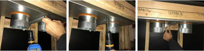
7 Remove the knockouts from the top of the fireplace. Use snips or diagonal cutters to snip the tab on the knockouts. Press on the far side away from the tap to pop the edge of the knockout up.
