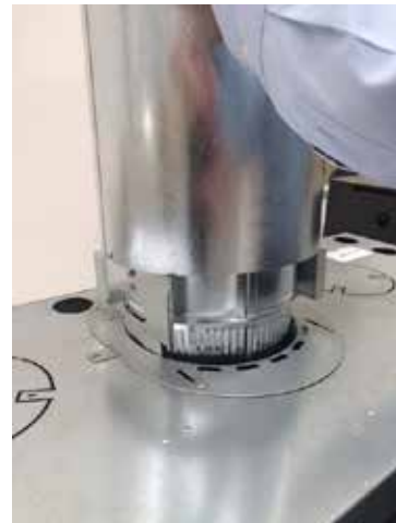
5. Air cooled bracket and pipe fitted to unit. The outer casing of the flue (10") must be raised 75mm above the zero clearance box.
