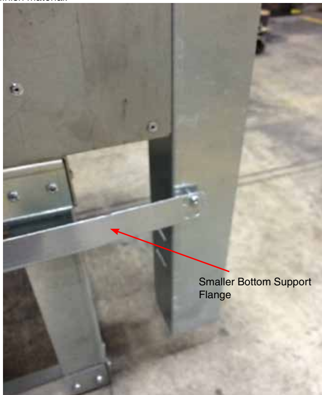
Support strip installed with slotted side on unit. The slot allows the movement of the support strip to be adjusted depending upon thickness of finish material.
