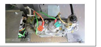
7. Make the gas line connection, bleed the gas line (if applicable), start the heater, and thoroughly leak-test all gas connections and the gas control valve.
