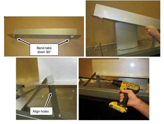
5 When finished the fireplace should be configured like the picture below.
