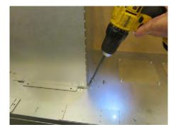
3 The (2) header standoffs are screwed down flat to the front edge of the top of the fireplace. On each standoff, remove the screw that is closest to the center of the fireplace (keep screw for reinstallation). Bend the legs at the perforations as shown below and attach the foot of the standoff to the top of the fireplace using the screw removed earlier in this step.
