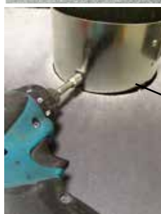
Duct collar secured with screws
