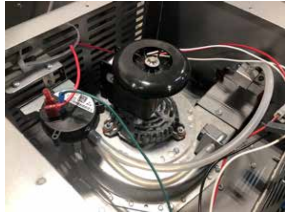
Pressure switch installed
