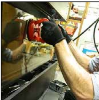
Handle glass with supplied vacuum clamps
