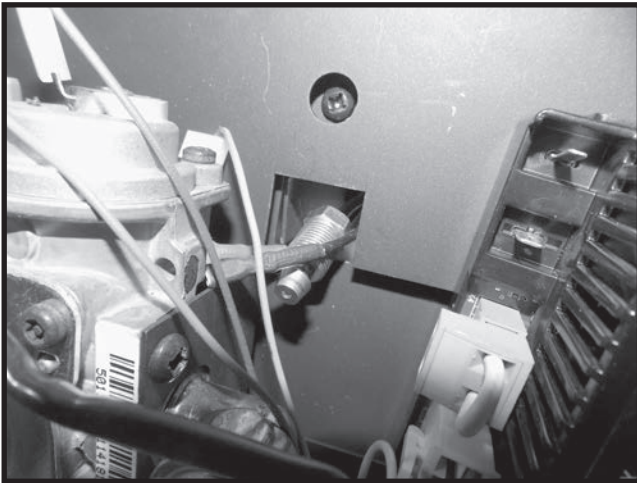
Figure 68: Square slot for insertion and removal of pilot assy.
