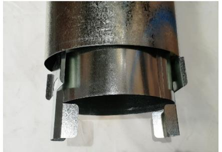
The 8" galvanised casing MUST be sealed with a heat resistant fire cement, like the flexible sealant Pioneer Fire Cement, around the top of the Zero Clearance box to stop heater air coming into the chimney chase cavity.
